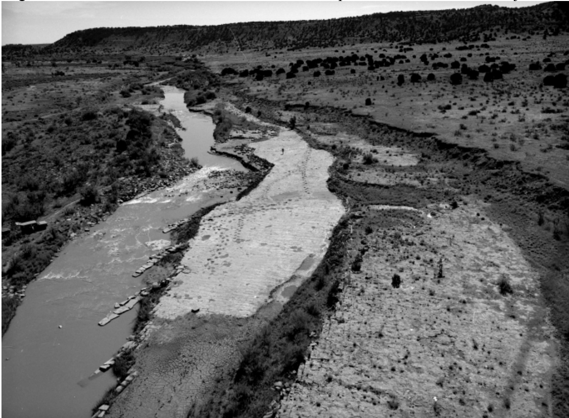
Picketwire Canyonlands, SE Colorado - Rock vanes used to protect dinosaur trackway. These structures were installed in 1998, and survived a 100 year event the following spring. Note the deposition and new willow vegetation taking hold in between the structures.
