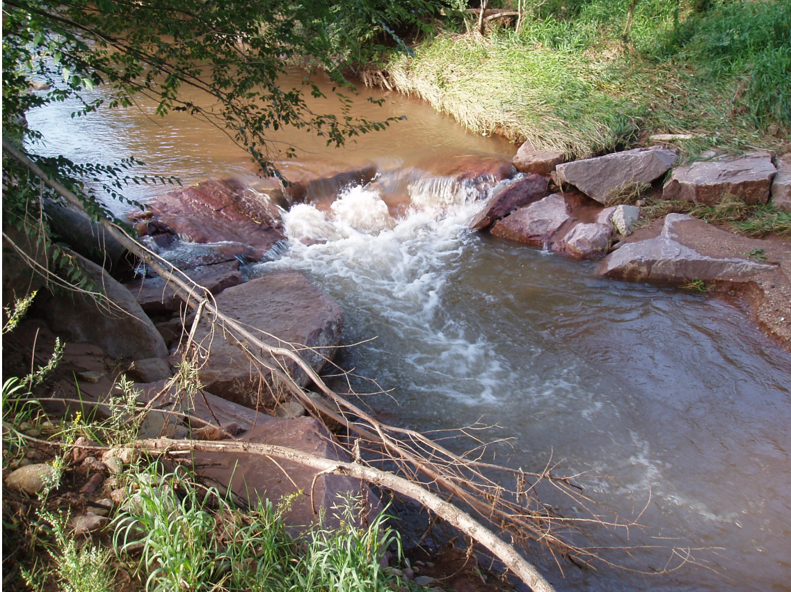
Cross Vane Structure on Fountain Creek below 21 st Street Bridge, El Paso County, CO.
