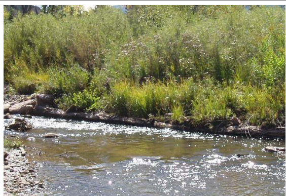
Photo 4: Log toe-slope stabilization of a stream
