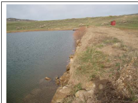
Photo 11: Lakeside Dam Face.
