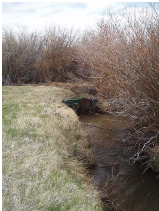
Photo 8: Existing Trophy Lake Diversion
