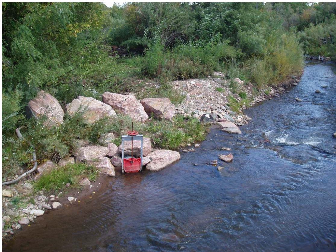
Photo 5: Typical 16" head-gate and culvert assembly, with a cross-vane immediately downstream. Cucharas River, Colorado..
